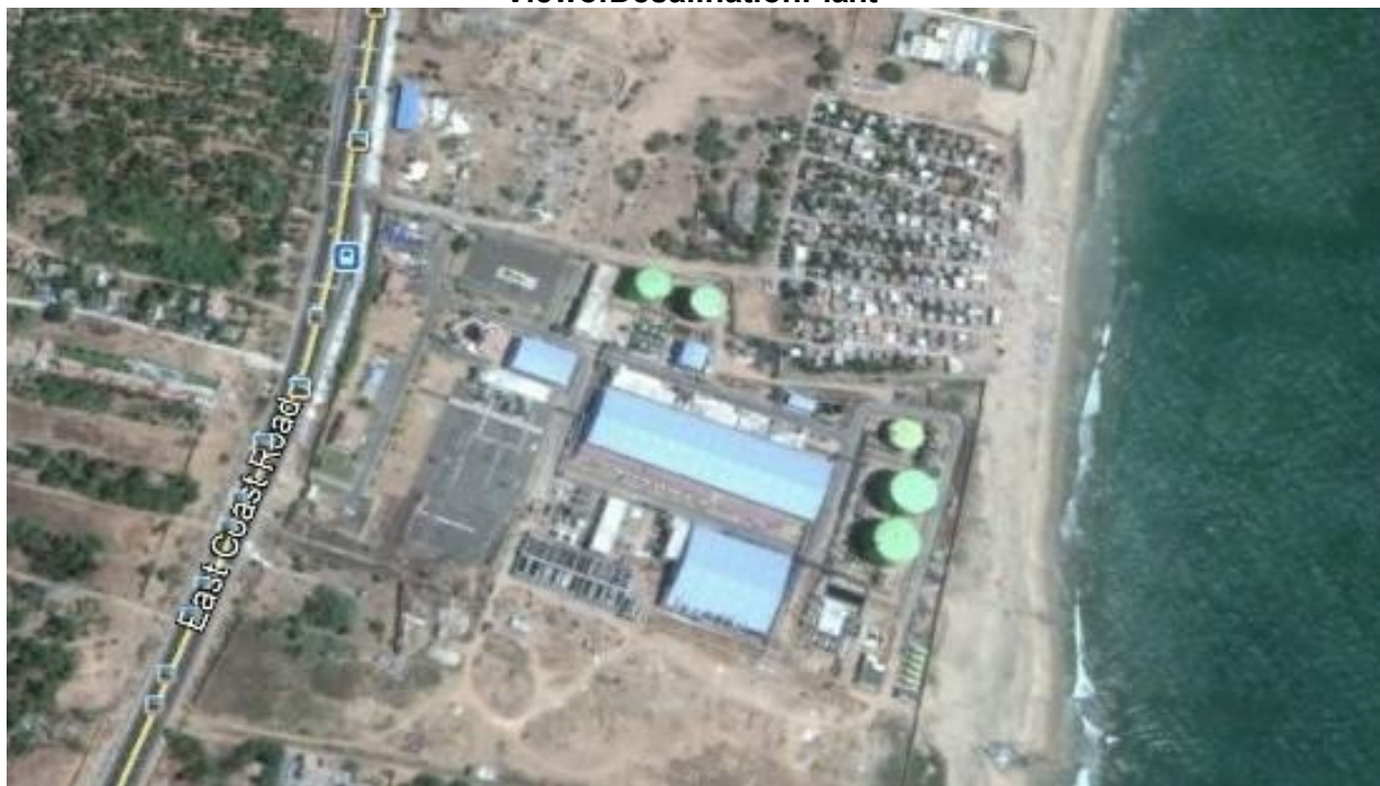
View of Desalination Plant
